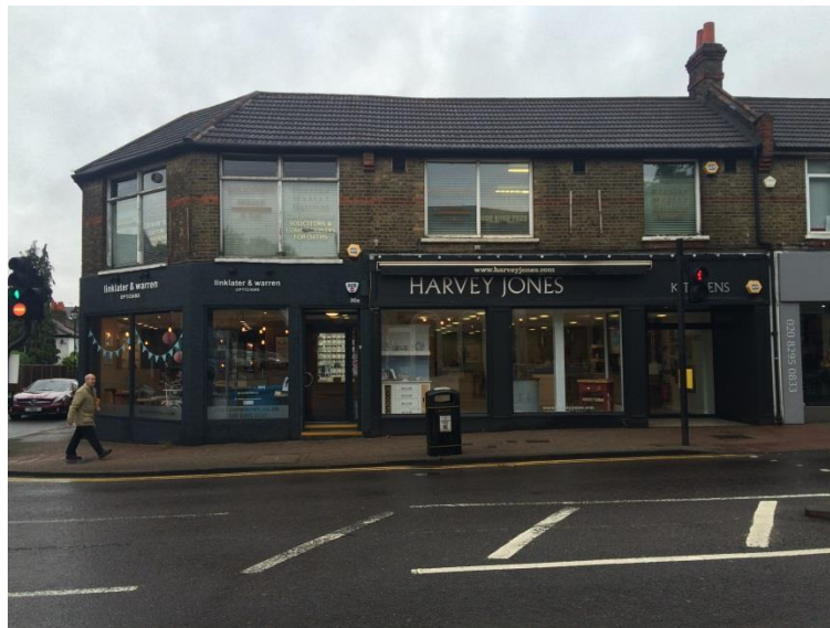
Fig.5 the premises of White & Bushell's Ironmongers, as it stands today on Chislehurst High Street, Chislehurst, Kent.
